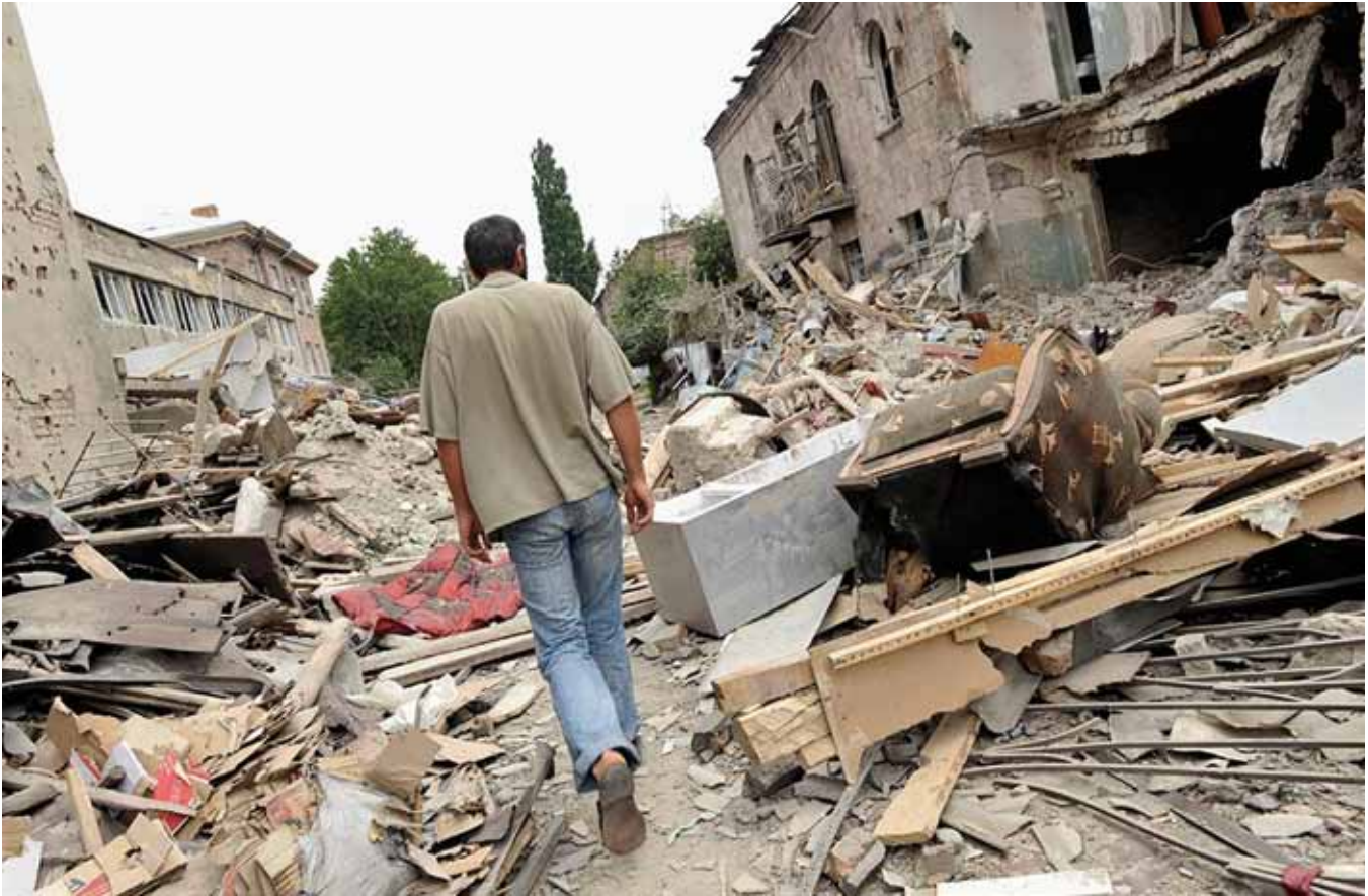
Bombarded Khakhutashvili Street, Kombinati settlement, Gori.
