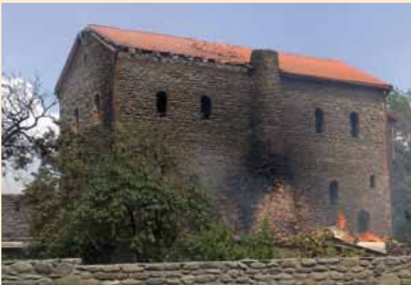
Building of Nikozi Eparchy damaged during the bombardment.
