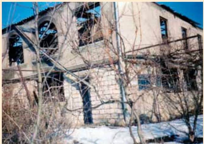
Bombarded village Ksuisi, December 2008
